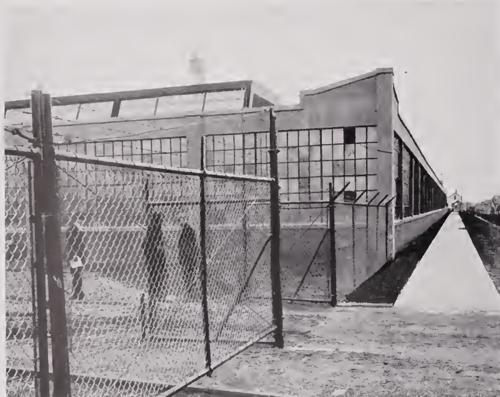
STEEL FENCING PROTECTS THE PROPERTY
